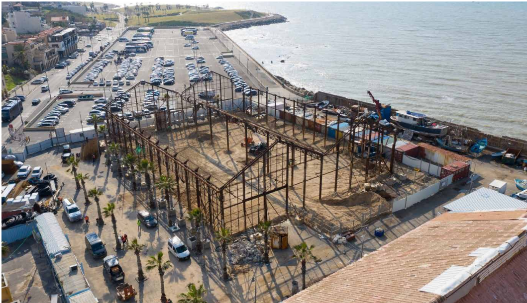
FIG. 6.18 Aerial view of the Jaffa Port redevelopment in progress, showing the skeletal remains of the historic port hangars during reconstruction. Source: Atarim Group
