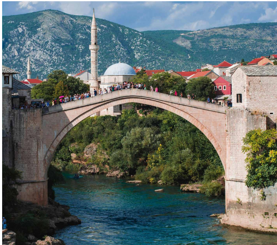
FIG. 2.1 The Stari Most bridge after reconstruction; Photo credits: Robert Dan
