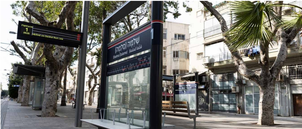
FIG. 6.14 The completed LRT station along Jerusalem Boulevard in Jaffa reflects the integration of contemporary transit infrastructure within a historic urban landscape through the preservation of mature Ficus Sycamore trees. Their incorporation into the final design followed nearly three years of advocacy efforts led by environmental activists, local residents, and civil society groups, highlighting the role of public participation and environmental consciousness in negotiating between urban modernisation and heritage preservation; Source: NTA Metropolitan Mass Transit System Ltd.
