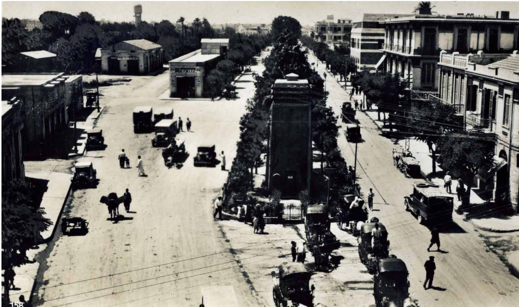
FIG. 6.11 The Jaffa Electric Company's secondary power station was inaugurated in 1923 on King George Boulevard, (later renamed Jerusalem Boulevard). Despite its historical and associational value to the city, as the first power station, it was demolished in 2007 without consultation or preservation efforts, marking loss of early-20th century industrial infrastructure in Jaffa. Photo courtesy: Tel Aviv Municipal Archives; Source: (Neiman, 2018; Groag, 2024)
