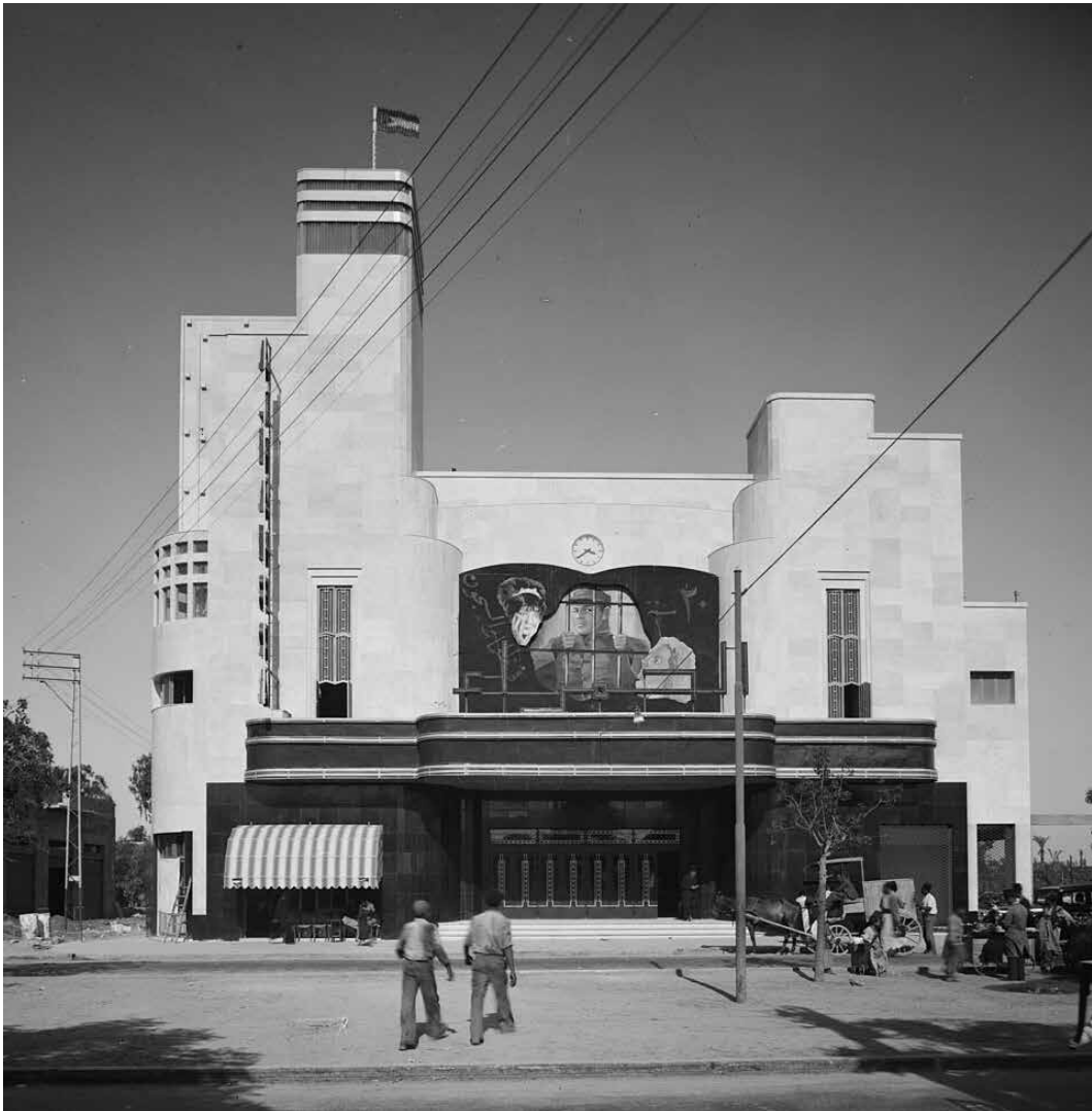
FIG. 2.10 Alhambra Cinema, an Arab cinema and cultural center in Jaffa, Jerusalem Boulevard 1937; Source: Matson Collection, Library of Congress. (Groag, 2024)
