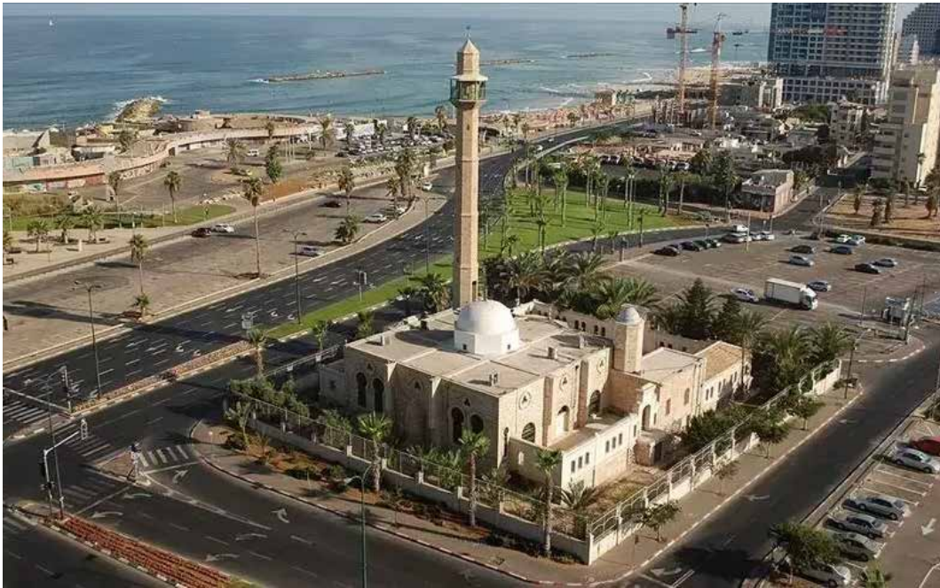
FIG. 5.16 Built by the empire's Governor Hassan al-Basri Aljabi in 1914, Hassan Beg Mosque; The mosque was spared during the destruction of Manshiyah in the 1948 war due to religious connotations. Later, it was proposed to be sold off as real estate to convert to a shopping mall, a move which was objected Jaffa Muslim Community. Currently, it is actively used for religious purposes, and has also seen the reconstruction of the minaret, taller than the original one. Source: The Daily News
