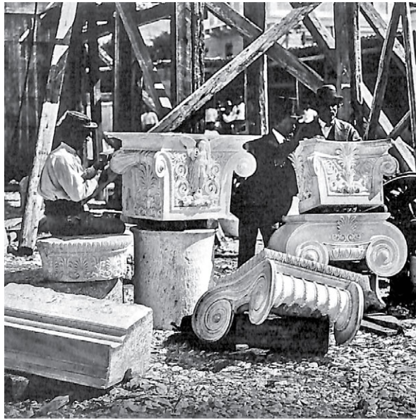
FIG. 1.16 Marble parts during the construction of the Academy of Athens. Photograph, ca. 1872–73. Τσίλλερ-Χάνσεν Αλληλογραφία, 1859–1890 [Ziller-Hansen Correspondence, 1859–1890].
