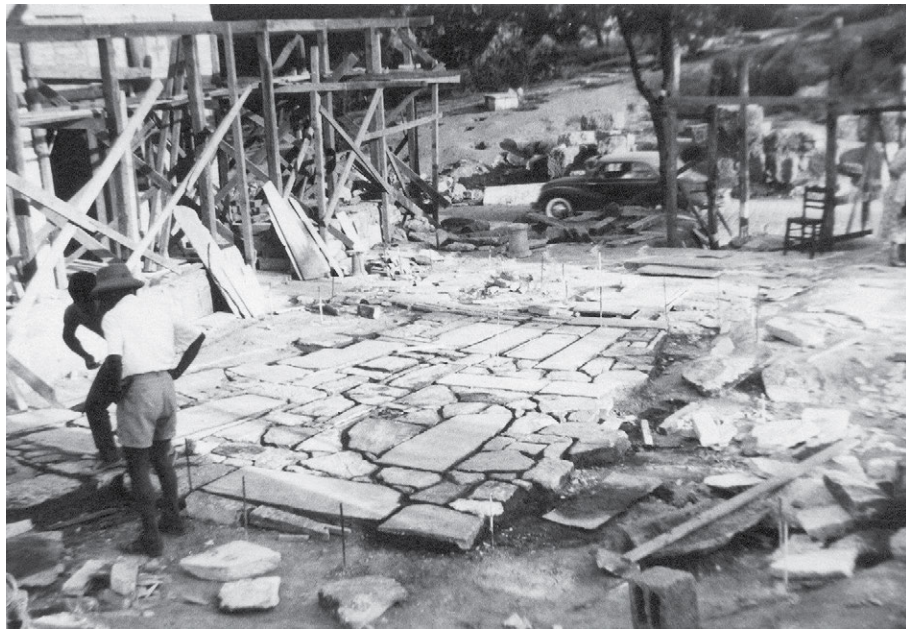
FIG. 2.11 Philopappou Hill pathways under construction, Athens. Photograph, ca. 1956. From Doma .
