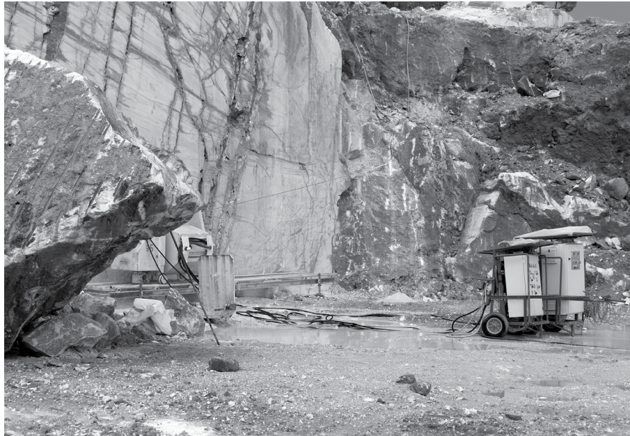
FIG. 3.2 Diamond wire cutting at Mount Pentellicus. Photograph by the author, 2025.
