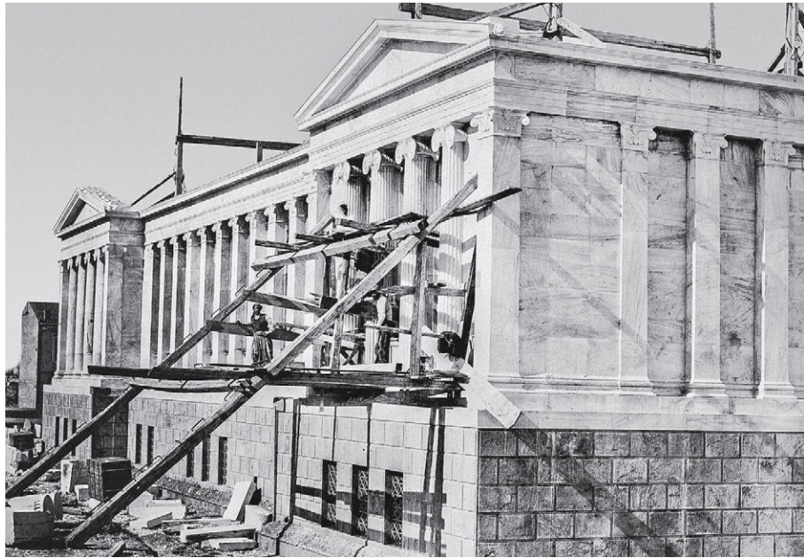
FIG. 1.13 East facade of the Academy of Athens under construction. Photograph, 1874. Τσίλλερ-Χάνσεν Αλληλογραφία, 1859–1890 [Ziller-Hansen Correspondence, 1859–1890].
