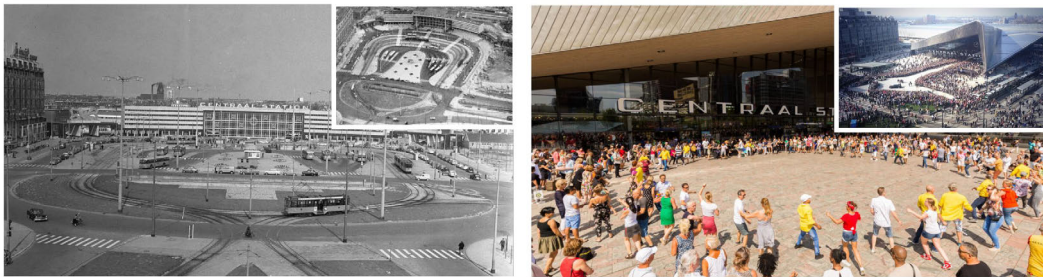
FIG. 6.13 The previous and the current Rotterdam Central Stations. (Sources: left-large— commons.wikimedia.org ; left-small— internaathetposthuis.nl ; right-large— tropicaliente.nl ; right-small— west8.com )
