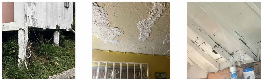
FIG. 3.8 Examples of damaged elements (A) damaged concrete piles; (B) patched concrete ceiling; (C) damaged wooden rafters.
