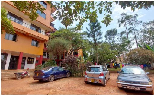
FIG. 6.21 High-end Rental Housing: Exterior and Parking Facilities, Kikoni.
