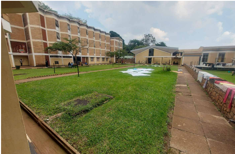
FIG. 4.10 Mitchell Hall Courtyard.
