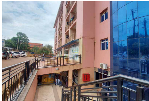
FIG. 5.36 Symbolic Landmark: New Nana Hostel (high-end facility with clinic and restaurant), Kagugube.
