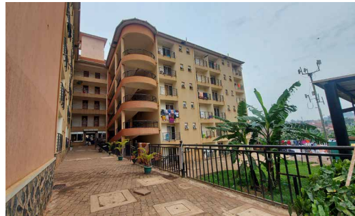
FIG. 6.18 Laundry-scape: Balcony Drying at Student Hostel, Kikoni.
