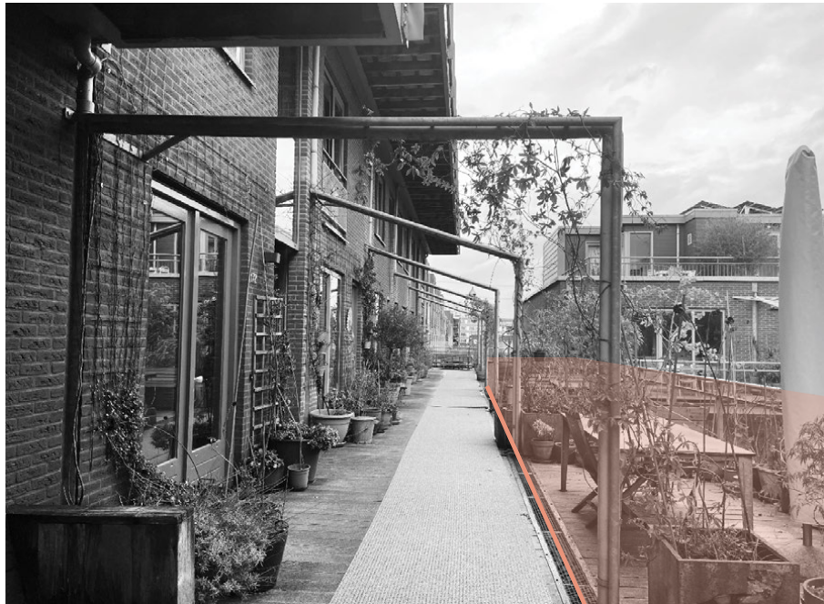
FIG. 5.19 Clarifying private and shared boundaries in Vrijburcht, where rainwater pipes mark the threshold between individual outdoor areas and the gallery's circulation area.
