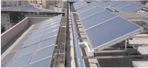
FIG. A.2 Double-glazed flat plate collectors (Mugnier et al., 2017)
