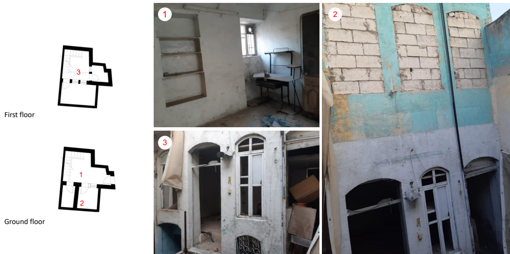
FIG. 6.2 The documentation for the traditional courtyard house (Type 1), cadastral number 1430, located in the Al-Aqaba neighbourhood, includes an AutoCAD-drawn plan and photographs of the interior façade and the room. The structure has been altered by returnees; Photo (2) illustrates the closure of openings using building blocks.
