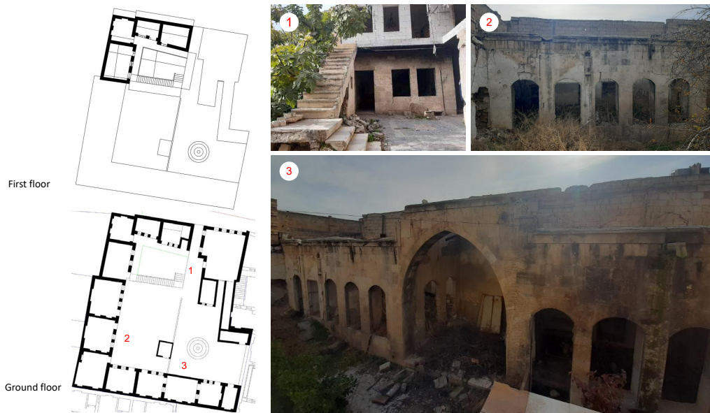
FIG. 6.5 The documentation for the traditional courtyard house (Type 4, with two courtyards), cadastral number 1520, located in the Al-Aqaba neighbourhood, includes an AutoCAD-drawn plan and photographs of the interior façade. The house has been partially destroyed; Photo (1) illustrates a new floor added by returnees.
