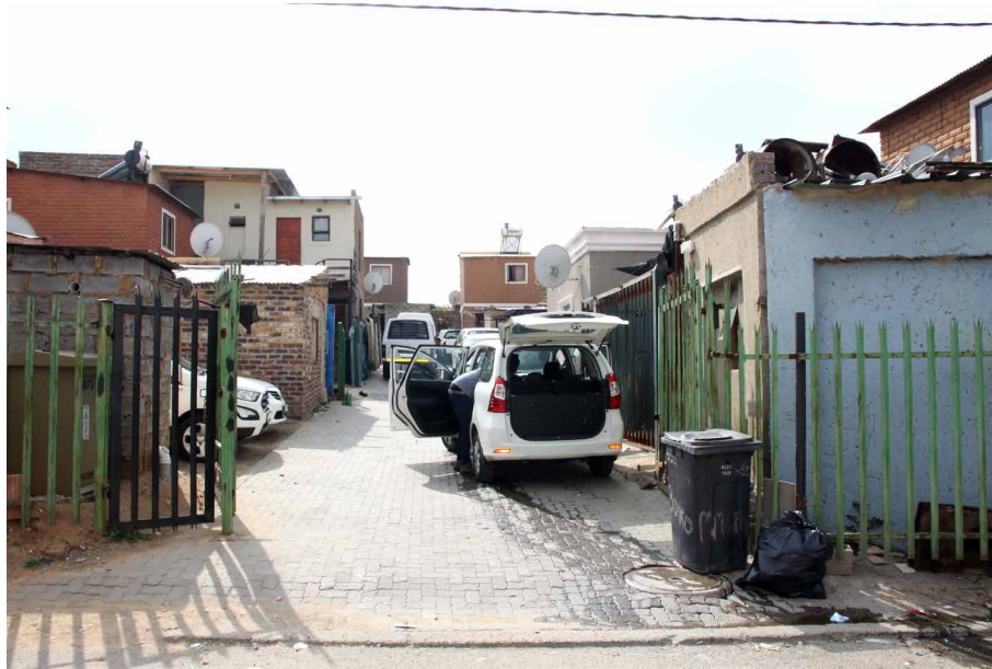
FIG. 2.13 Image of Cluster in Phase 2 K206 depicting incremental extensions over time, palacade fencing, multiple materials and extension types clearly depicted within the photograph (Source: Author(2021))
