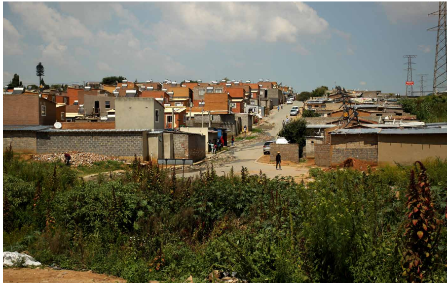
FIG. 2.11 Image looking at phase 4 of the K206 Development. Houses on the left are Type 1 houses, and houses to the right of the road are Type 2 and Type 3 houses as indicated in Figure 2.12 below. Brown brick finish is reminiscent of original housing, and in most case plastered walls or non plastered stock brick communicates incremental expansions (Source: Author(2021))
