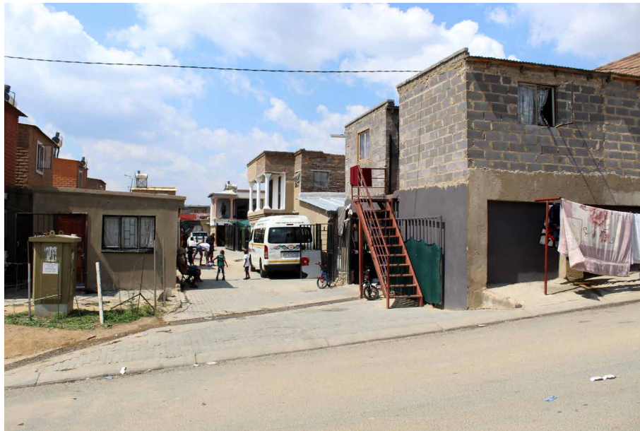
FIG. 2.12 Image of K206 cluster in Phase 4 depicting incremental extensions over time, double storey extensions more popular as a form of incremental extension in these depictions. (Source: Author(2021))
