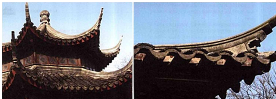
FIG. 4.14 Nen Qiang Fa Qiang (left) and Shui Qiang Fa Qiang (right) (Construction technology of Suzhou Xiangshan faction 苏州香山帮营造技术)
