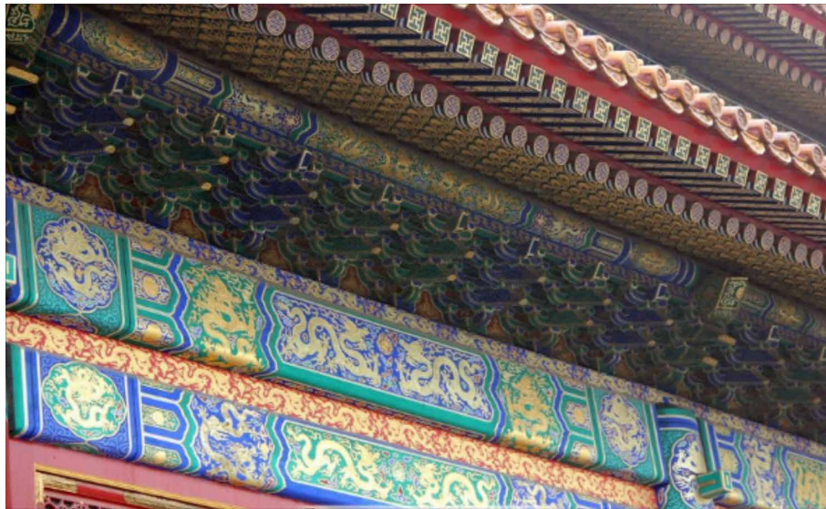
FIG. 3.6 Chinese traditional architectural elements: Dougong (wooden brackets) and Caihua (colour painting) (www.photophoto.cn)
