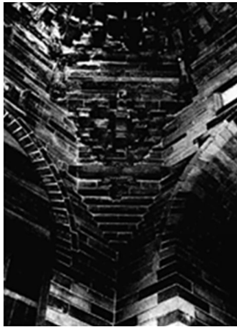
FIG. 4.12 The inner structure of the Beamless Hall of Suzhou: the connection between the circle plane of the vault and the square plane of the wall (Sicheng Liang)
