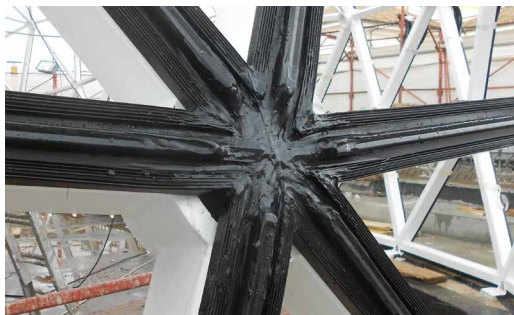
FIG. 2.30 Single-layer cut and joined joint Ex-Unione Militare (Image courtesy of Guido Ranieri Da Re)
