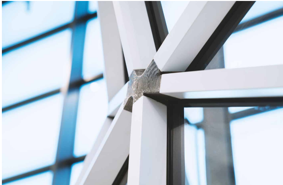
FIG. 6.4 Detail view of additively manufactured structural node in freeform façade for Glasstec 2022 (Image courtesy of Jansen AG)
