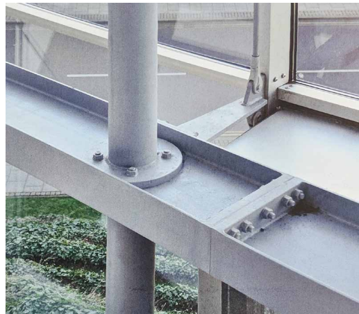
FIG. 2.17 Structural node of the Sage at Gateshead façade – a geometrically optimal surface divided into quad panels) constructed using traditional steel framing methods (Image source: [47])
