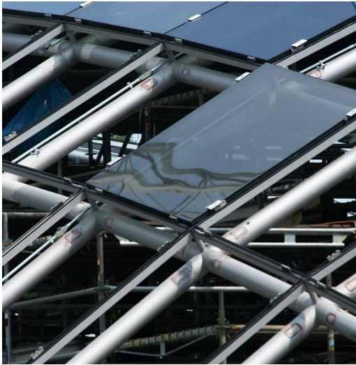
FIG. 2.21 Offset support of Mansueto Library (Image source: [122] (CC BY-SA 2.0))
