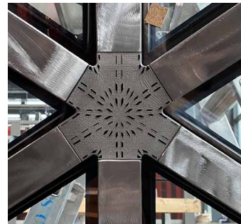
FIG. 6.25 PBF-L node in first full-scale mock-up assembly (Image courtesy of Jansen AG)
