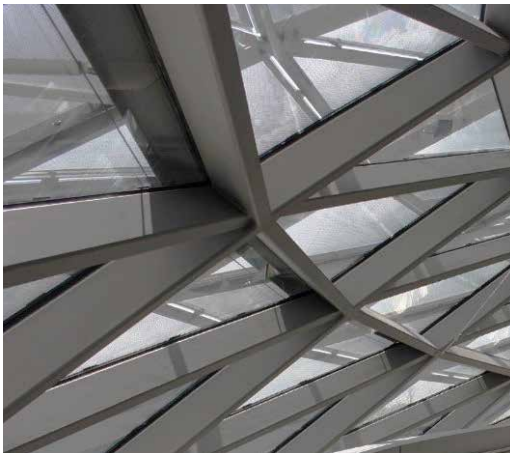
FIG. 2.16 Directly welded node from BMW Welt façade, a true freeform geometry requiring complex cutting and welding of profiles (Image courtesy of Frank Dinger)
