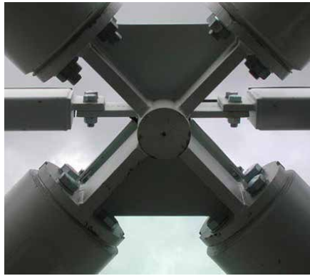
FIG. 2.9 Built-up node with end-face and splice connections from A2 Cockpit in Utrecht. (Image courtesy of ONL)
