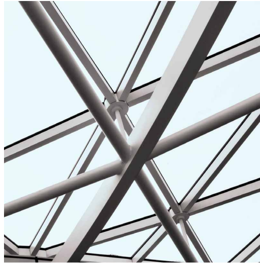
FIG. 2.22 Cylindrical node on steel structure of King's Cross Station. (Image courtesy of Barrie Tate)
