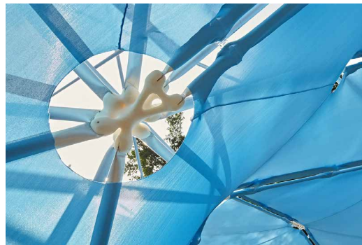
FIG. 3.6 3D Printed ABS node using FFF for aluminium pipe and lycra canopy. (Image source: [132])
