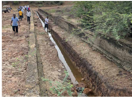
FIG. 4.4 A 500 m long drain discharges water from Umasar Lake toward the qanat system of 24 wells (left), of which two are depicted in the right image, to transport the water underneath a hill toward Hamirsar.
