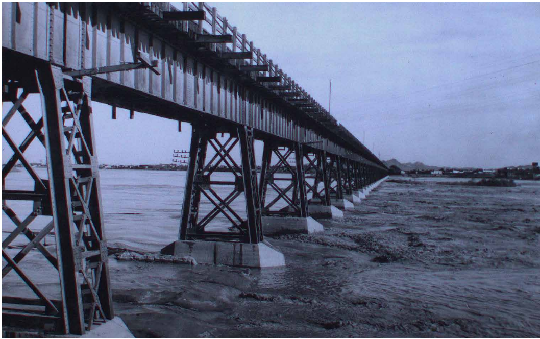
FIG. 4.17 The Railway Bridge Over the Karun: it is Built on the Foundation of the Ancient Dam.
